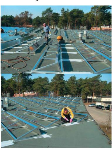
The adhesive tensile strength values determined by the Braunschweig Materials Testing Centre Germany are many times the holding forces for wind suction load required by DIN 1055.
